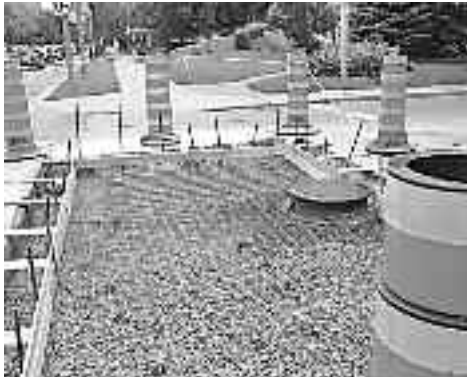
Left: A crosswalk at Sherbrooke and Lansdowne was redone with steel reinforcement mesh, seen August 22. The sewer rim appeared crumbled. Right: Deep transversal cracks appear on the crosswalk in this August 23 photo at the same location.
