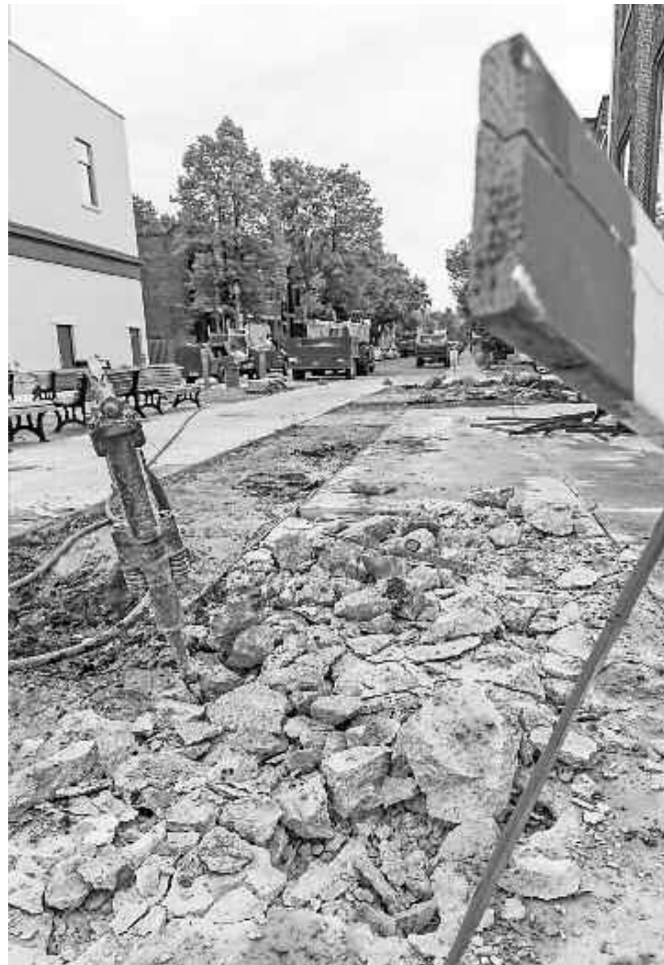
Pneumatic drills, picks and shovels were at work May 25 around 8 am at Prince Albert square to correct paving deficiencies before planting can take place.
