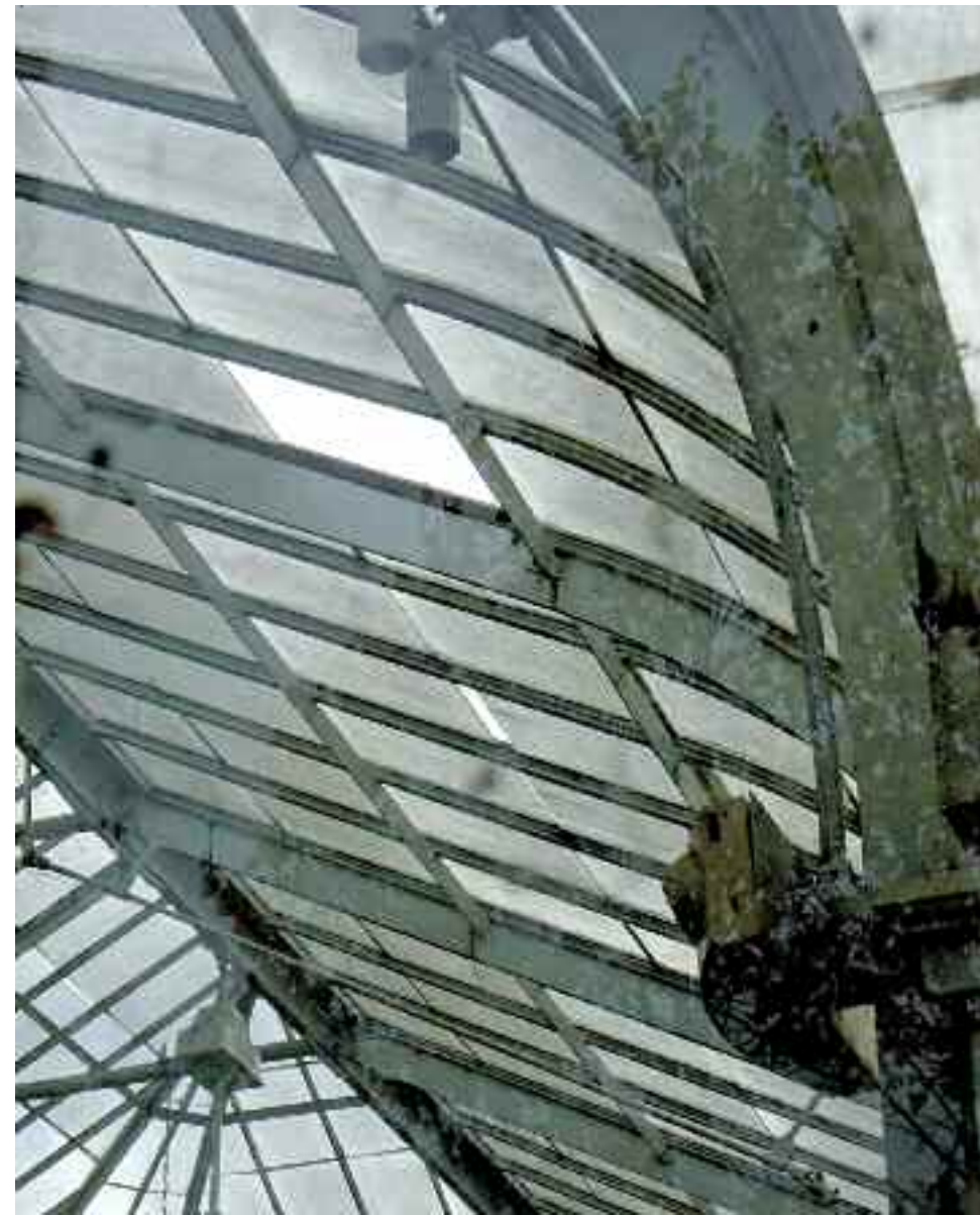
The fallen pane can be seen in the same row of overhead windows where several others are seen slipping October 16.
