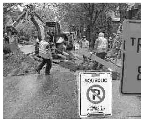
Another week, another waterline break. City workers repair a water main break on Argyle just below. Westmount Ave., on the west side of Argyle, May 22. A city foreman told the Independent that the water main was relatively new but a rock, moved about by thawing and freezing of the earth, punctured it, causing a near flood in a neighbouring home. The break was repaired by the evening. Photo: Robert J. Galbraith
