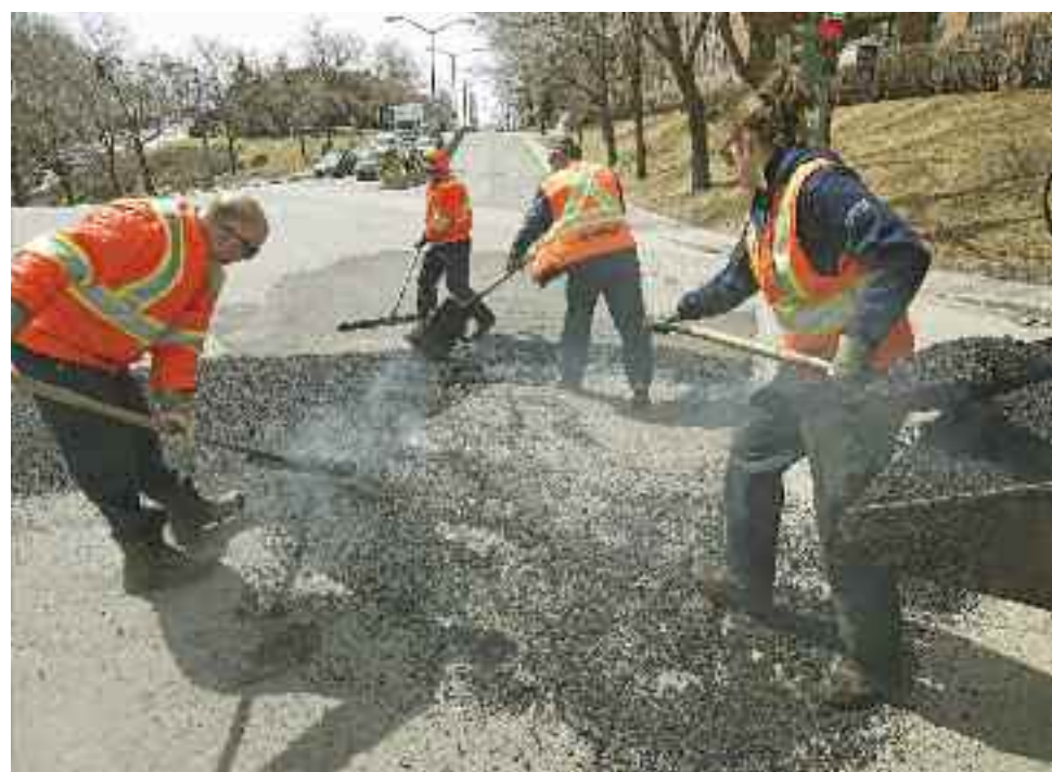
A Westmount Public Works crew takes advantage of a beautiful spring day to fill potholes and cracks in the city's road system at Lansdowne and St. Catherine streets, April 11.
