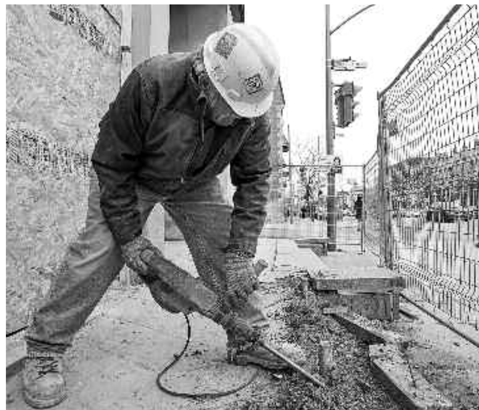
Construction foreman Yves Raymond of Emcon Construction uses a hydraulic drill-hammer to remove a section of the entrance ramp at the former post office at the corners of Sherbrooke and Prince Albert, March 27. The vacated building is being prepared for its new occupant, Lululemon Athletica.
