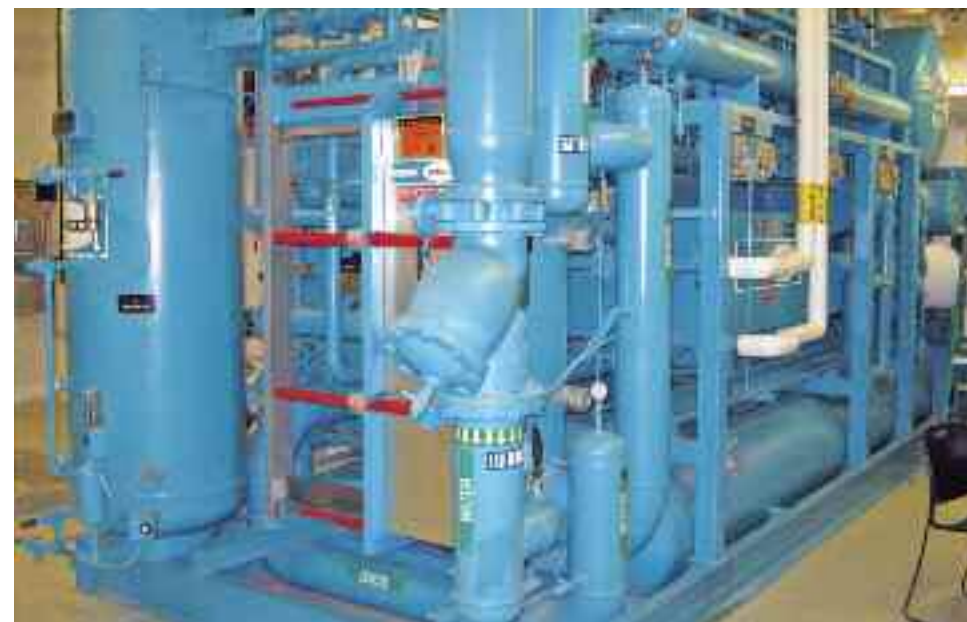
Three ECO Chill compressors maintain ice on the WRC's two rinks
