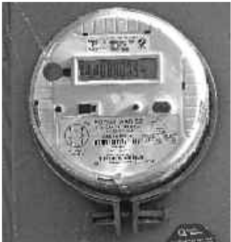
Hydro-Quebec’s RF “smart meter,” transmits electrical consumption directly to billing offices. It is a Landis + Gyr “Focus” model.
