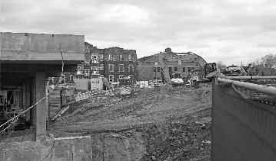
The pools’ changing rooms level was visible on April 10 and useable for two workers at left, but the dirt to the south has to be removed to get it to the same level. Also, the pools themselves have to be excavated one layer lower.
