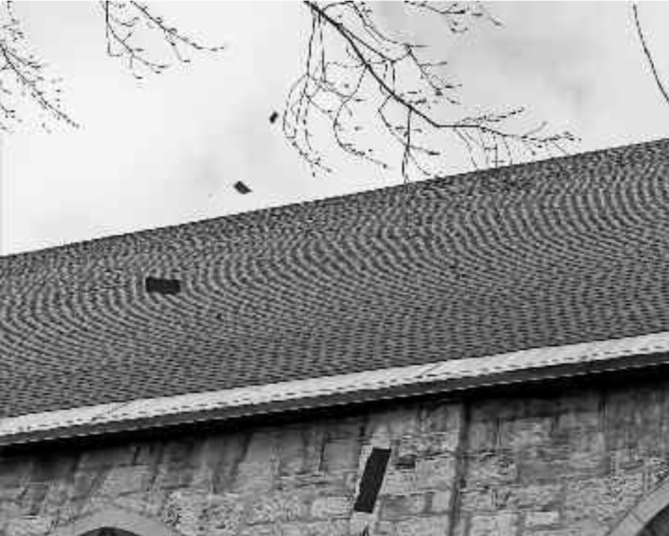
With wind speeds up to 100 km/h, shingles were ripped off large sections of the roof of Westmount Park United Church January 31. This photo was taken around 2 pm.
