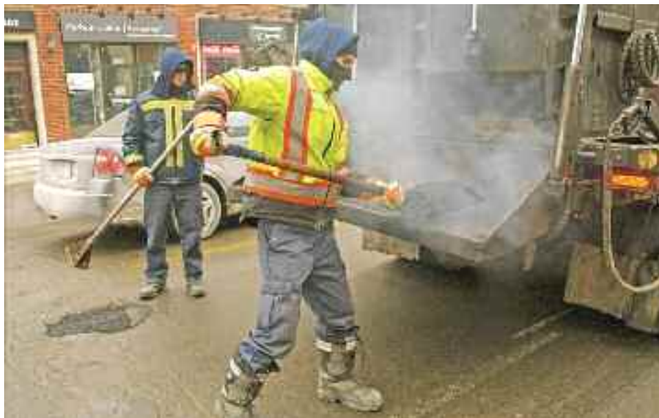
Public Works employee Marco Brunetti shovels hot, steaming asphalt from the back of a city truck as colleague Justin Cavanagh Jackson pounds it down into potholes on St. Catherine St. January 24. See story, p. 15.
