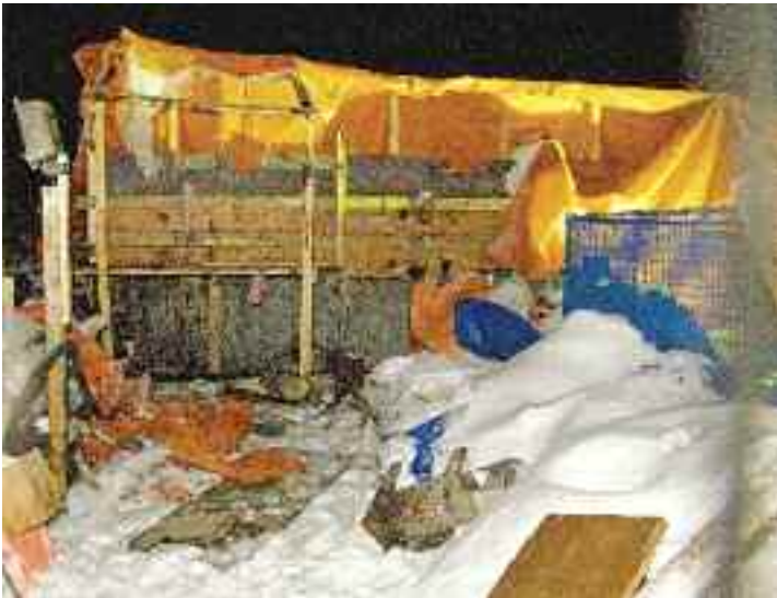
Minimal damage was caused at the northwest corner of the new Westmount arena/pool construction site on de Maisonneuve near the corner of Lansdowne the evening of January 20. An overturned heater ignited a plastic cover tarp. The fire department put out the blaze.
