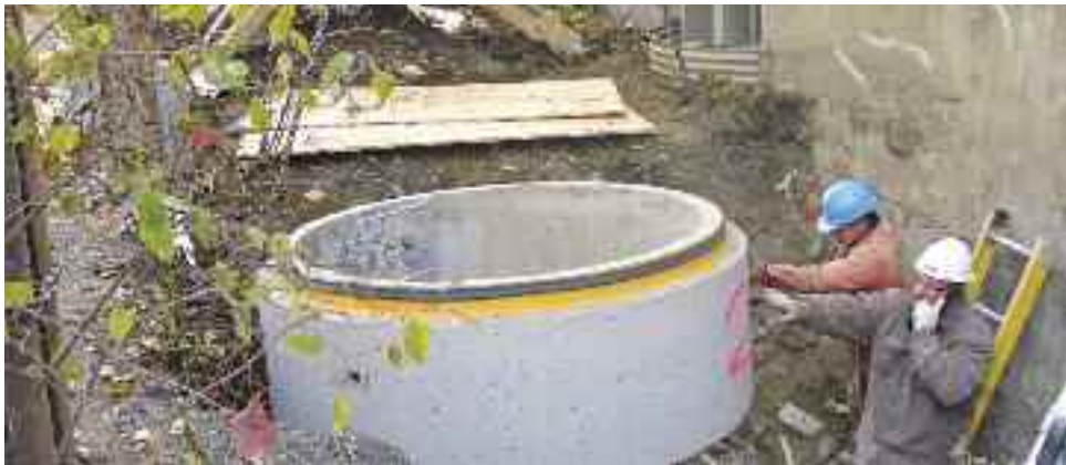
At the southeast side of Westmount Park Church, workers lower a concrete section of an access chamber to an old manhole November 8 as part of a project to cap a century-old pipe draining into the site of the Westmount recreation centre.
