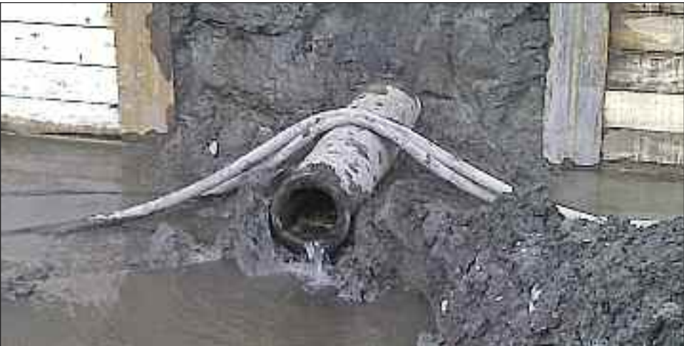
Water leaks from 12-inch abandoned sewer line September 19, where it passes from the north under de Maisonneuve.
