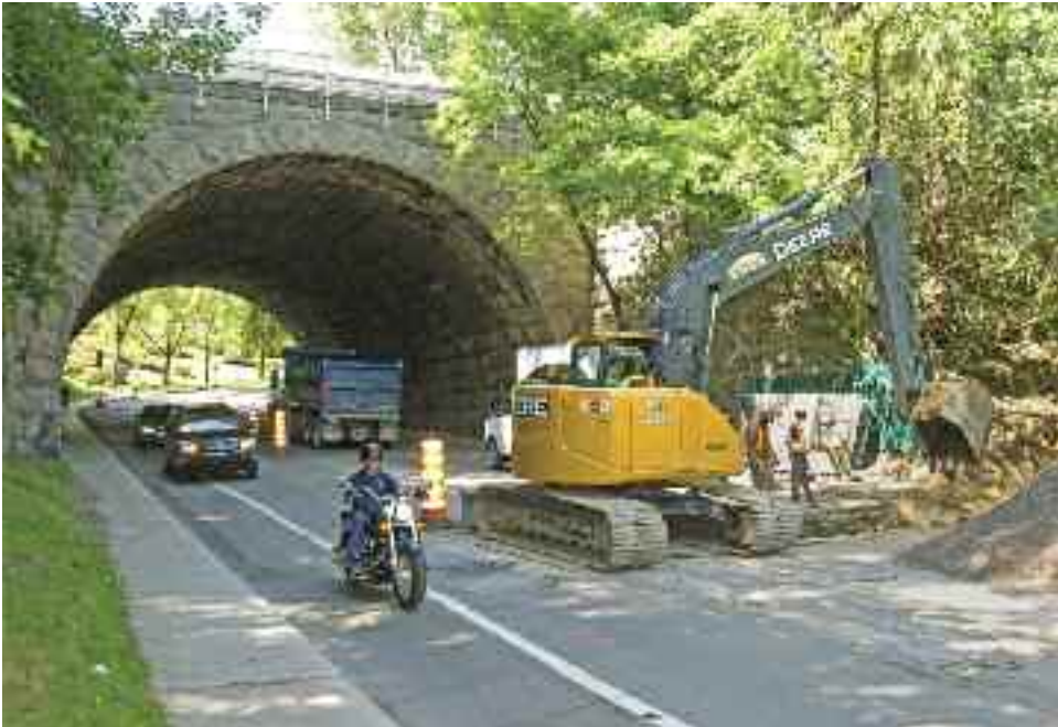
Contractors work on laying and connecting drainage piping from the CP railway bed above the Glen railway overpass to the main sewer line that runs under the Glen roadway. Andrew Duffield, now former assistant director of Public Works, explained that, “water percolates through the soil of the rail bed and spills down the side of the overpass onto the roadway. So this will alleviate the spillage.” The work started August 1 and was completed by August 3. During the work, north to south traffic was restricted to one lane.
