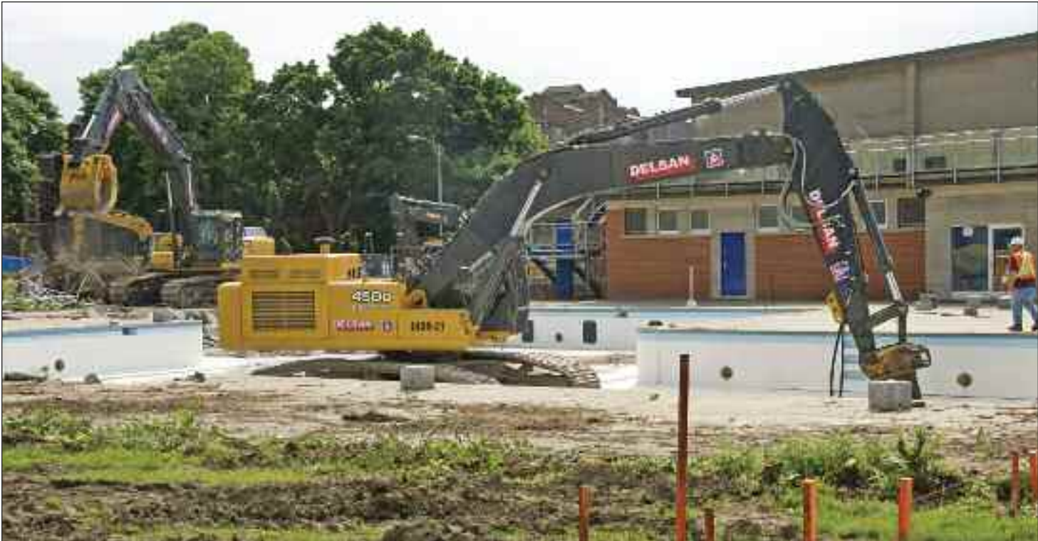
Hydraulic excavators start the demolition of the Westmount pool, May 28. The two machines positioned themselves over and in the pool area to better demolish it. By the end of the day, there was no trace of the pool, just a hole filled with earth and stone, and a pile of rubble. Demolition of the arena started the following day.
