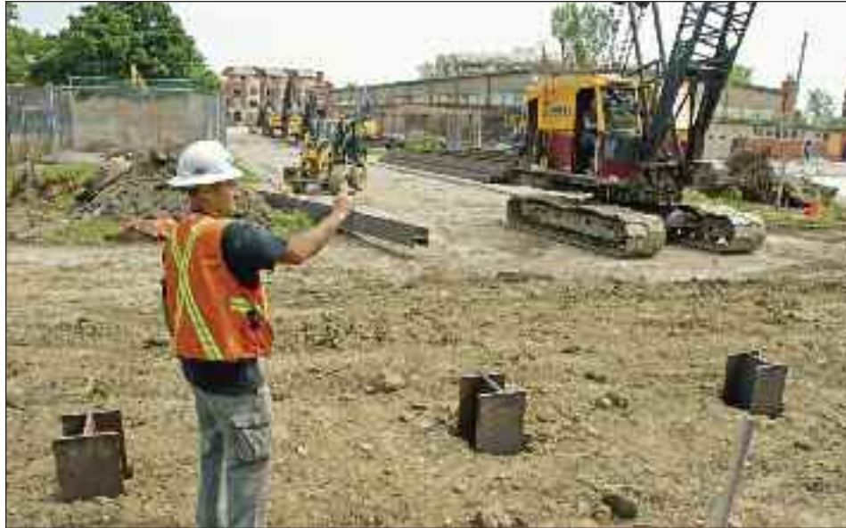
A worker at the Westmount arena and pool project construction site takes a photo of the site and the progression of steel piles being driven into the earth by a pile driver.
