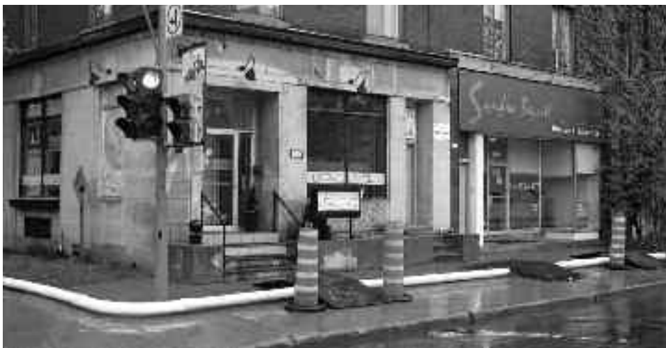
A temporary pipe, pictured here on May 8, has been set up on the northeast corner of Grosvenor and Sherbrooke to maintain water during a water main rehabilitation. The work is scheduled for completion in mid-June, with road repairs targeted for a week later. The work is being done for the city by Sanexen.
