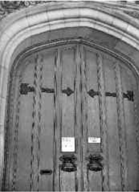
From the exterior, the front doors of city hall now push inward to enter. In order to reverse their swing to push open from the inside in compliance with fire regulations, the entire door frame assembly must be moved forward because of the arched top.
