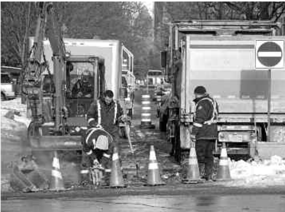
Contractors TranSelec Common work to repair a blocked underground Bell Canada conduit on de Maisonneuve Blvd. at the intersection of Claremont Ave. January 18. One of the workers cuts the asphalt pavement with a cutting tool while a back hoe with a pneumatic bit waits to pulverize concrete to expose the pipe containing the cables. Meanwhile, traffic was re-routed between Prince Albert and Claremont. The work was completed by January 21.
