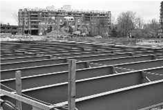
The steel roof structure gets built above the east rink.
