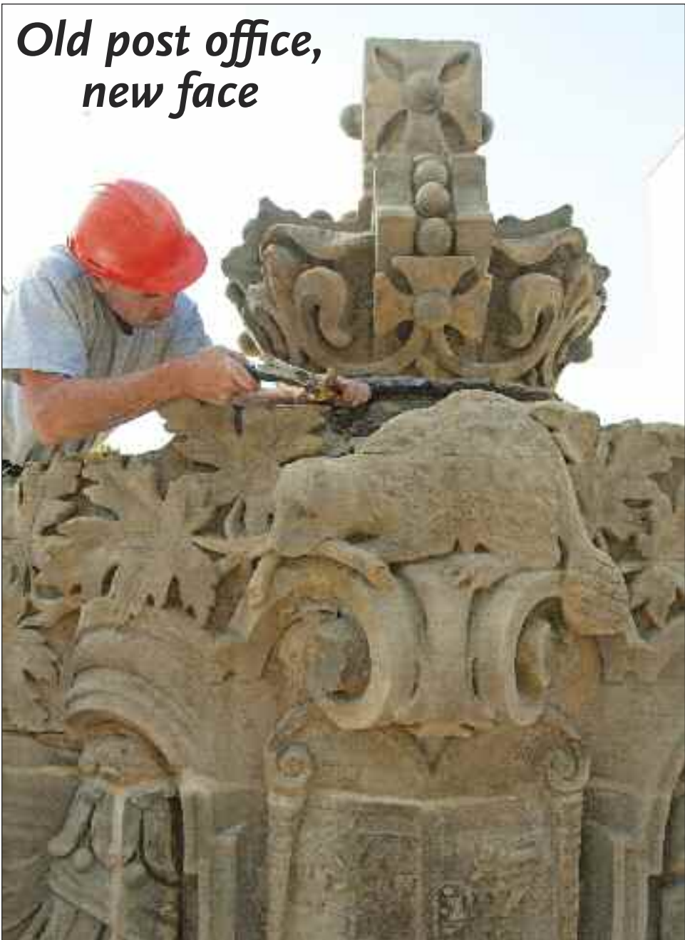
In preparation for the installation of copper flashing, a sheetmetal worker chips away at old roofing tar from the base of a yellow sandstone relief on the top of Westmount’s old post office building at the corner of Greene and de Maisonneuve on September 28. See p. 10.
