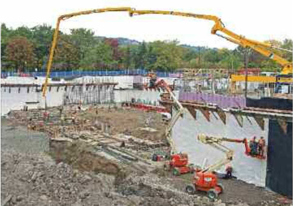
Westmount city councillor Patrick Martin told the Independent that concrete pouring began the week of October 1 at the new arena. Pictured here is concrete being poured via a pump and mechanical arm.
