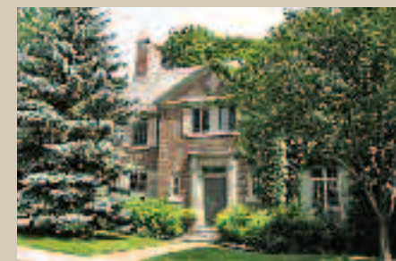
WESTMOUNT – 4302 Montrose $2,465,000 A traditional and refined exterior with all the right elements inside.
