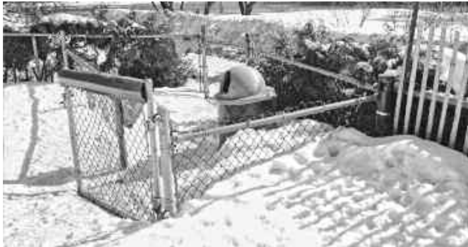
During an inspection of the Lansdowne dog run, an accumulation of snow seen next to a fence at the inner gate would allow dogs to effortlessly walk over the fence from the dog run's main area into the enclosed entrance section. Except for a minor ground clearance problem because of snow build-up, both gates appeared to be in working order.
