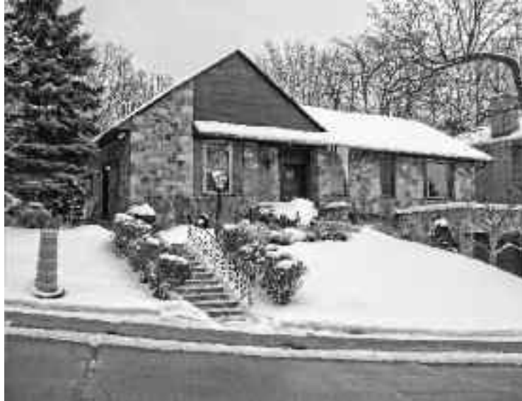
Existing bungalow at 28 Devon.
