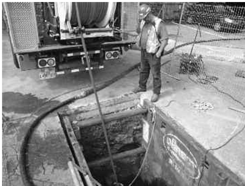
An Insituform Technologies worker power washes the water main under Prince Albert in preparation for the installation of a cured-in-place pipe liner.
