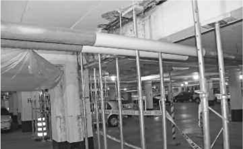
A photo of the second floor of 4300 de Maisonneuve apartment complex’s two-storey underground parking garage taken on May 23. The image shows plastic hanging from the ceiling, crumbling concrete, exposed rebar and some of the more than 400 poles scattered between the two floors.
