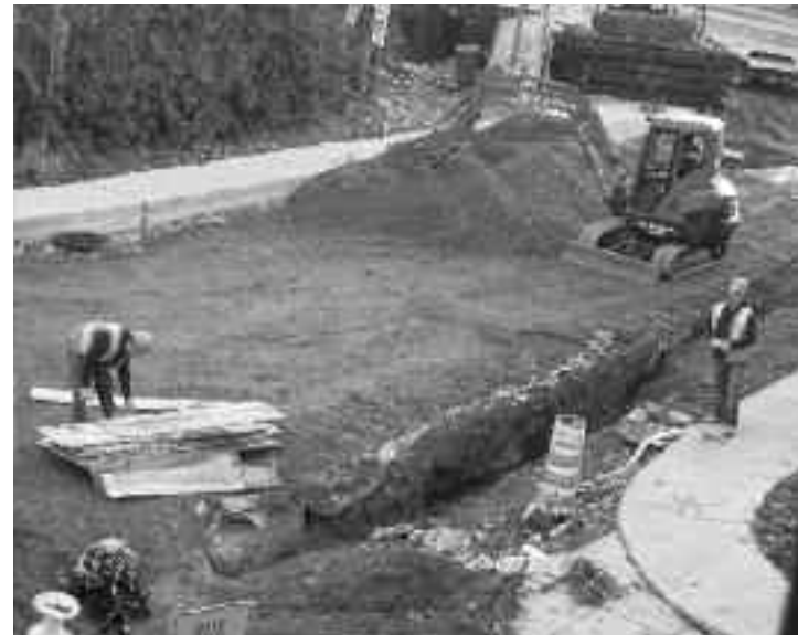
Bell contractors work on Prince Albert near York, November 16. The trench for Bell's conduits that was dug after the initial gravel grading was being filled in and was covered by the end of the day.
