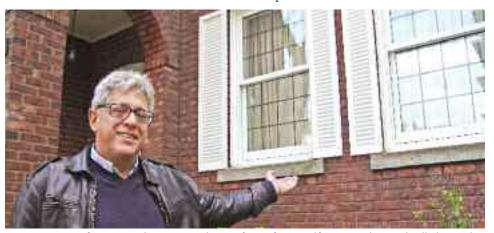
Martin Cooper of Martin Industries, standing in front of 244 Redfern Ave., shows a leadlight window replica that encases the lead strips inside the double glazed thermal unit.
