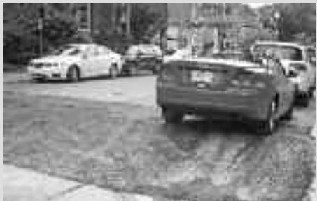
This temporary asphalt hillock protects a water pipe on Prince Albert just south of Sherbrooke, which will provide water to buildings when work begins next week on the water main between Claremont and Victoria.
