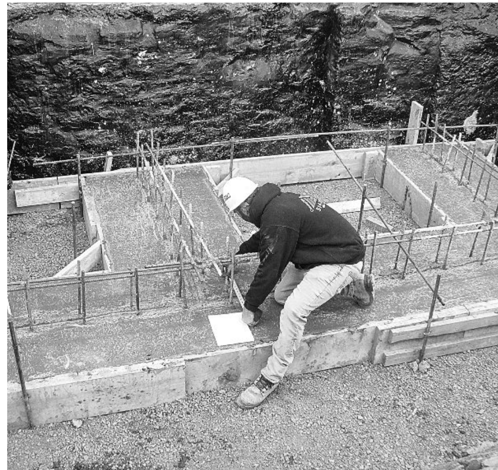
As seen September 24, preparation is under way for the new staircase at the entrance to Victoria Hall under the city's contract with PHLP Construction and Excavation.
