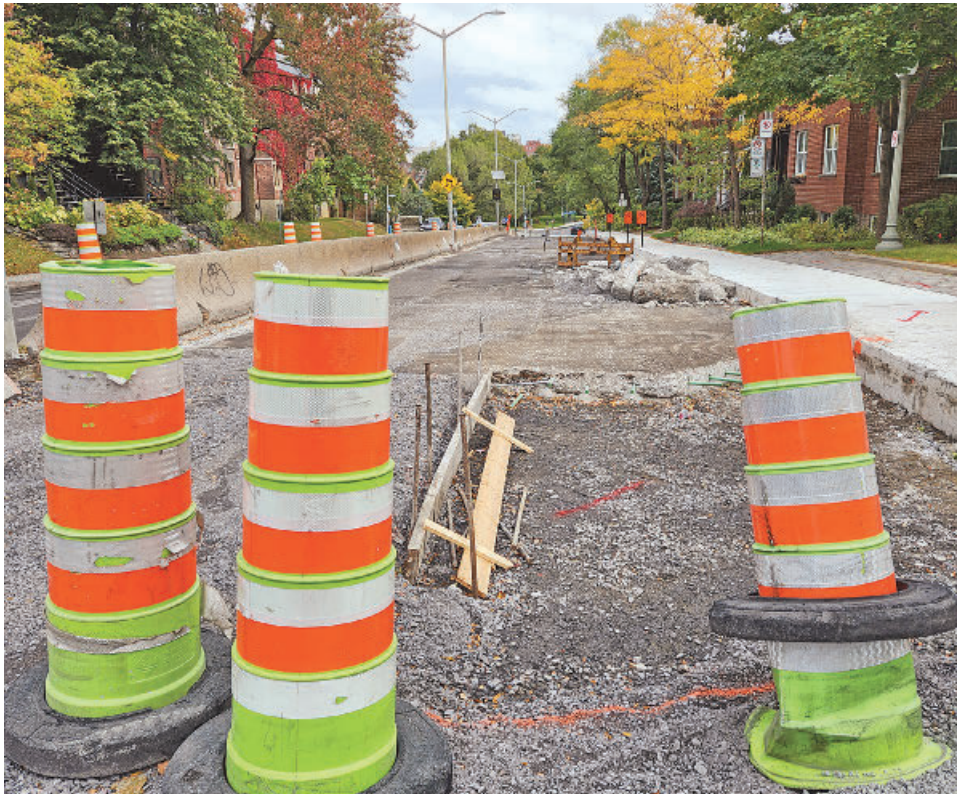
Looking east on September 28. During construction, St. Catherine remains two-way from Lansdowne to Victoria, but one-way (eastbound) from Claremont to Victoria.
