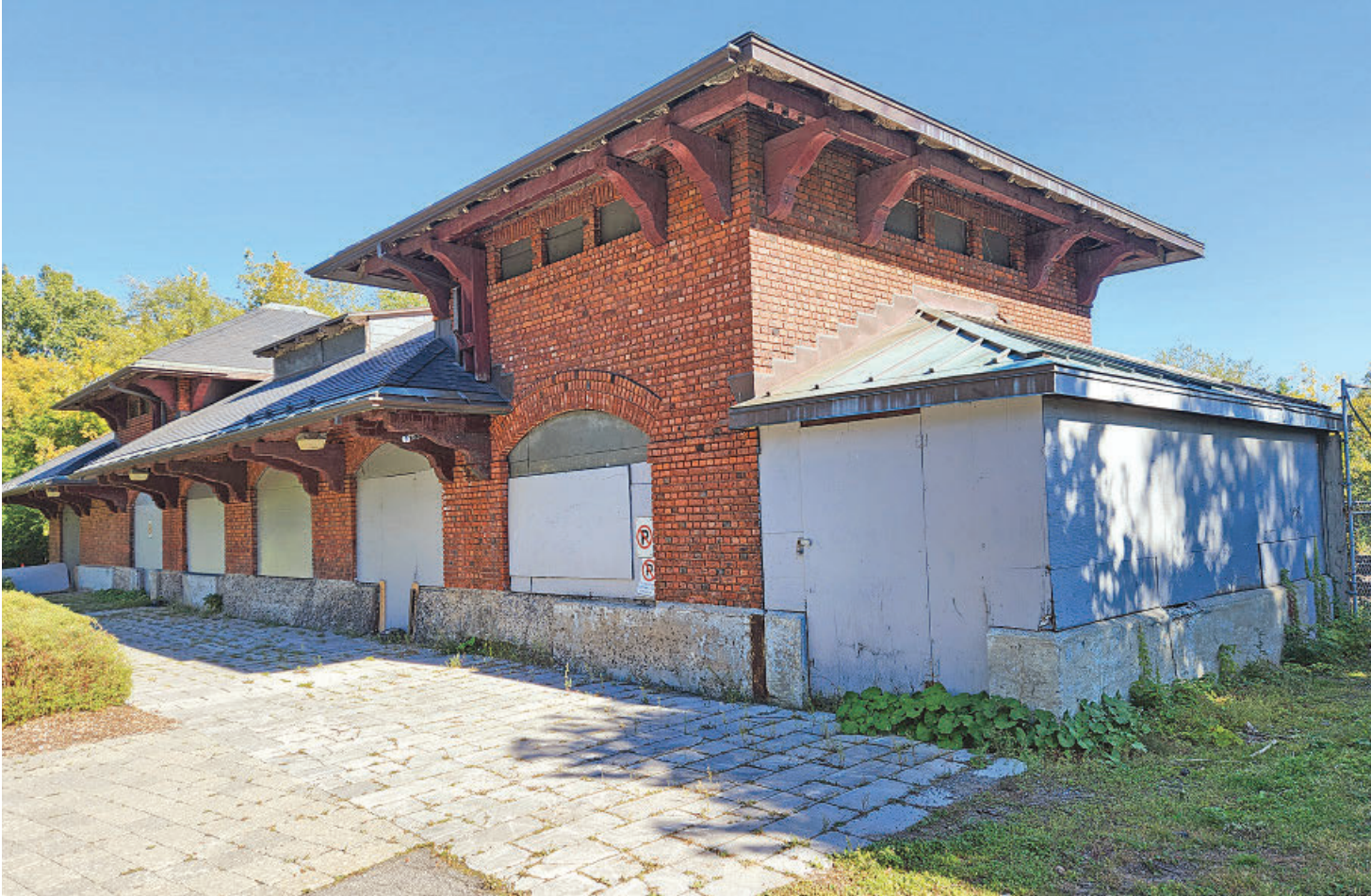
Looking southeast at the Victoria Ave. train station on September 24.
