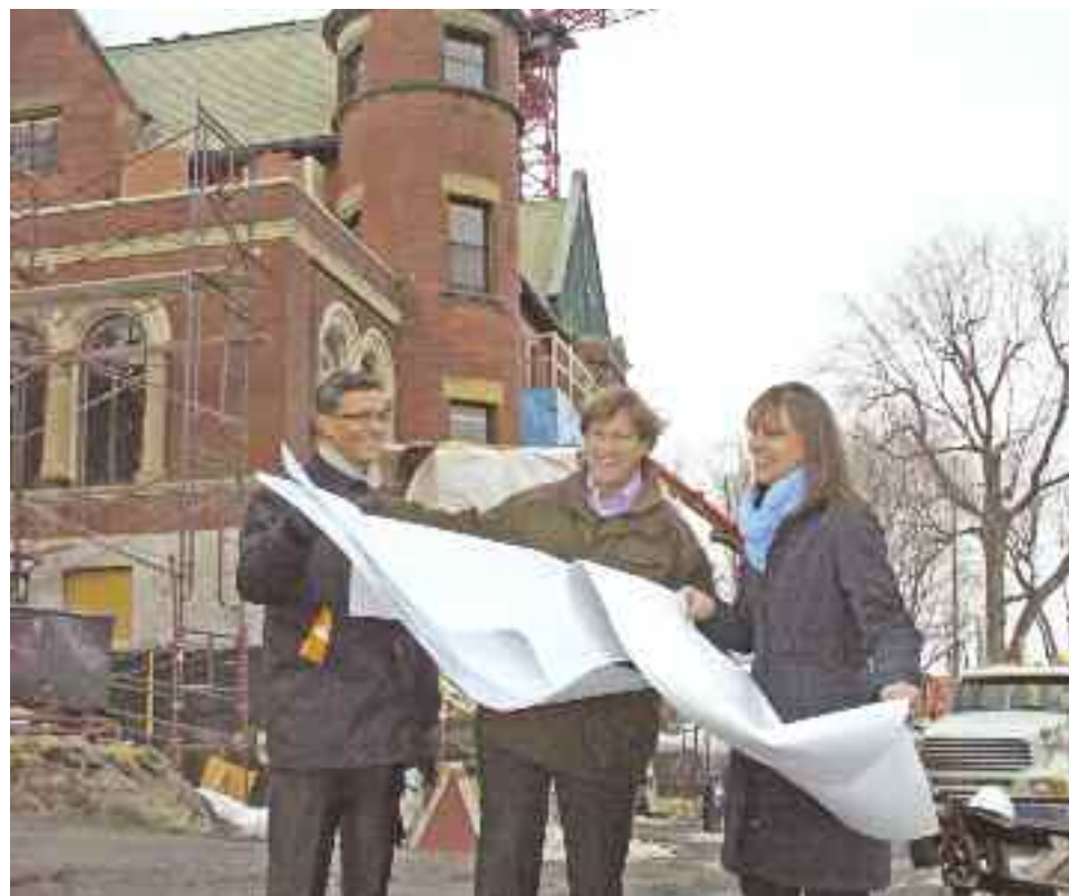
In front of the house, from left: Stephen Bronfman flanked by contractor Garry Garbarino (left) and architect Andrea Wolff.
