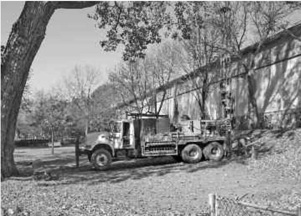
Lansdowne/St. Catherine dog run on October 31. Exploratory bore holes are being used to assess ground under and around arena.
