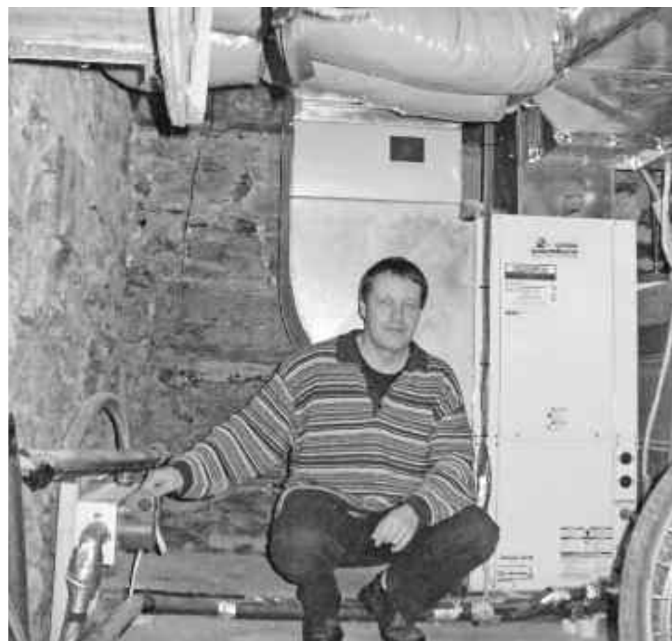
Paul Marriott explains how the ground heat enters the home (at left) to be pumped by the heat pump (behind him) through the basement ceiling ducts as a forced air system throughout.
