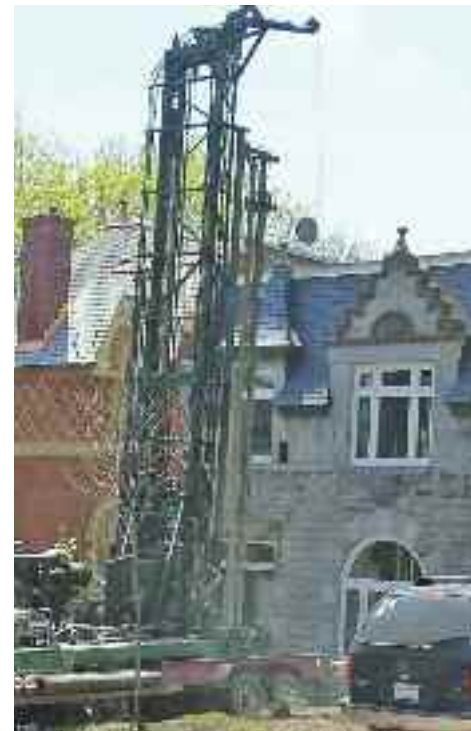
Drilling – not for oil but to avoid the use of oil. Black limestone gravel from the operation was spread along the alley and packed solid.
