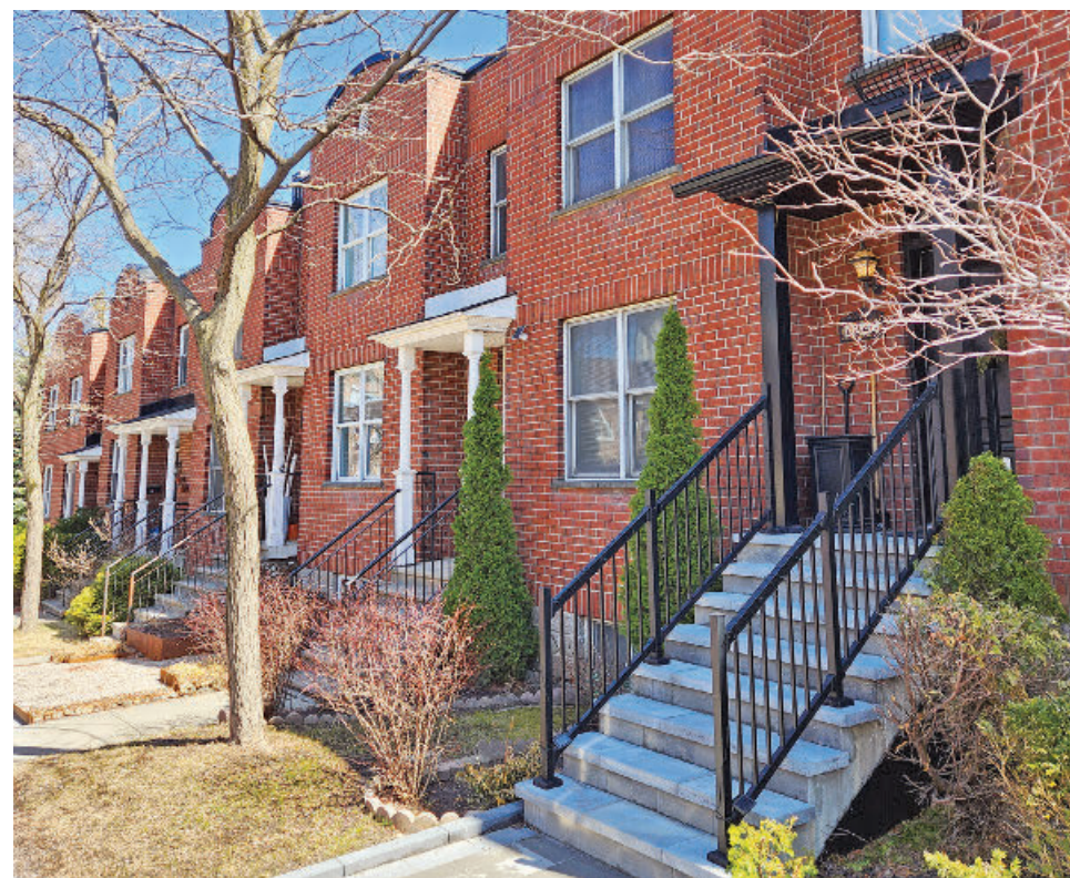
4840 St. Catherine St. is the house in the foreground with the black posts, as seen April 4.
