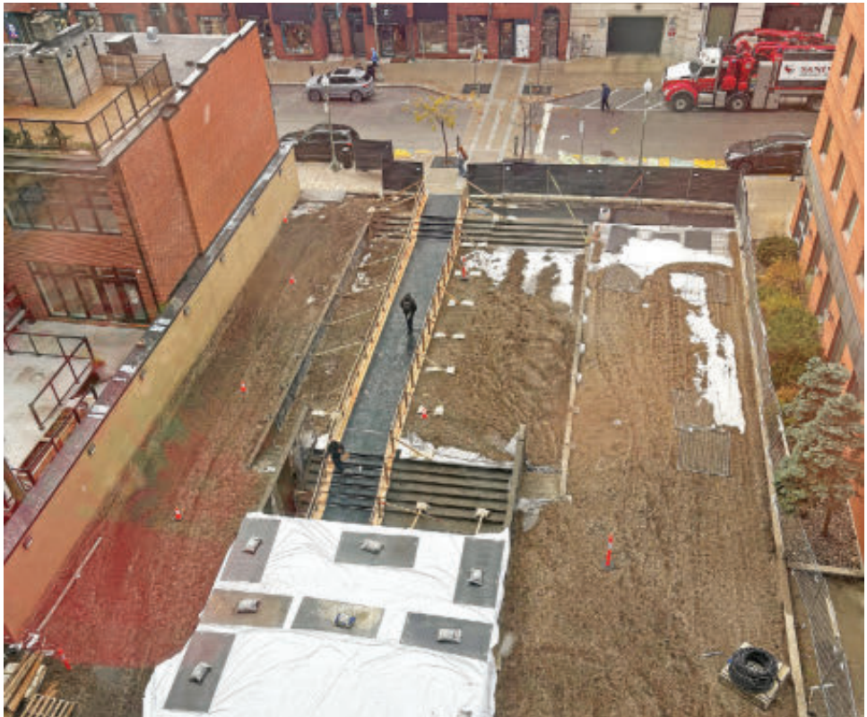
Temporary access to Westmount Square’s concourse and its tunnel to Alexis Nihon opened on November 27, as seen the same day. The area is the target of a major rejuvenation project (see October 21, p. SL-22, November 11, p. 10).
