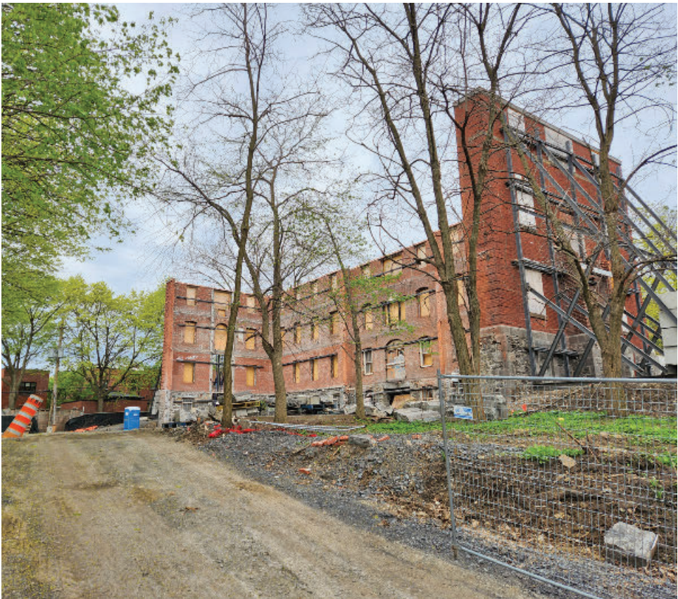
The demolition of 500 Claremont in order to preserve parts of the façade and build an apartment building continues, as seen May 8. Note the numerous, large counterweights to keep the shell balanced.
