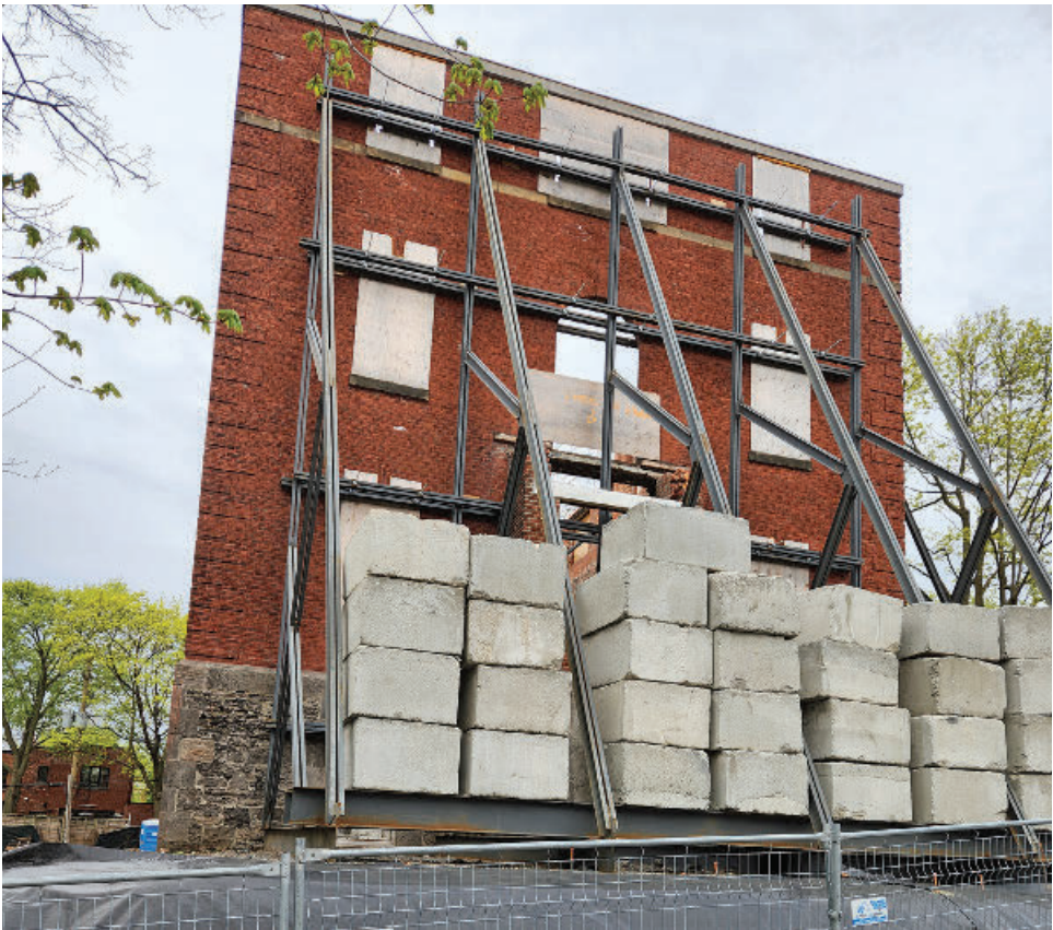
The demolition of 500 Claremont in order to preserve parts of the façade and build an apartment building continues, as seen May 8. Note the numerous, large counterweights to keep the shell balanced.
