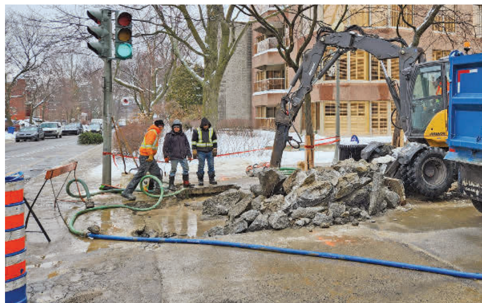
Workers repaired a water main leak on Victoria south of de Maisonneuve January 18, above, and then flushed the system via a hydrant on de Maisonneuve east of Victoria, below. PHOTOS: INDEPENDENT.
