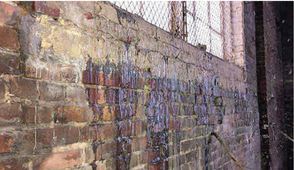
Photos from an inspection report by Underwriters’ Laboratories showing the Hillside Lane wall (the east façade), which is to be dismantled due to the level of corrosion of its six metal columns and the deterioration of its bricks.
