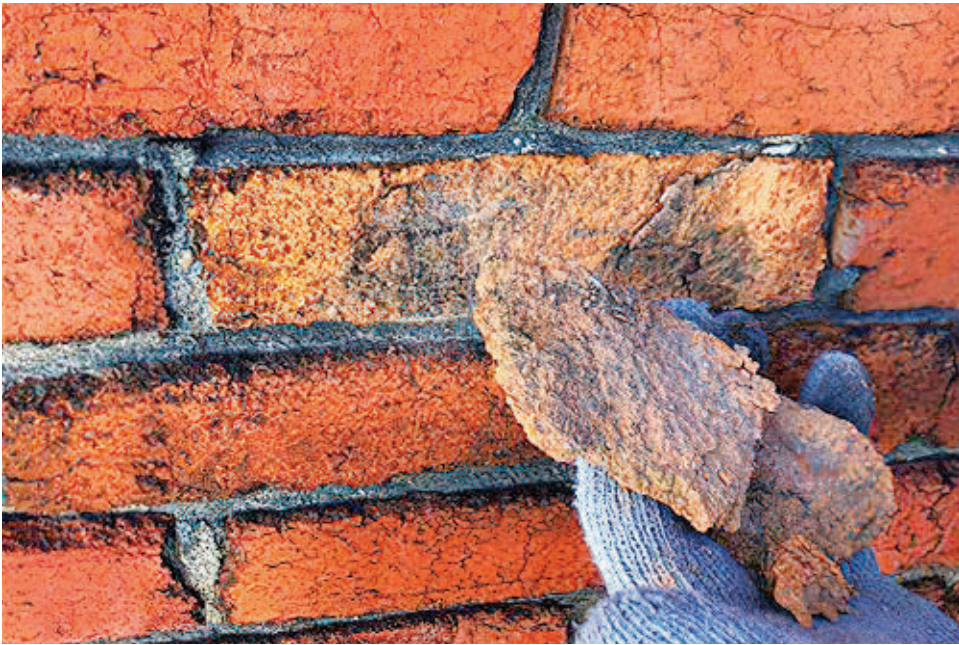
Photos from an inspection report by Underwriters’ Laboratories showing the Hillside Lane wall (the east façade), which is to be dismantled due to the level of corrosion of its six metal columns and the deterioration of its bricks.
