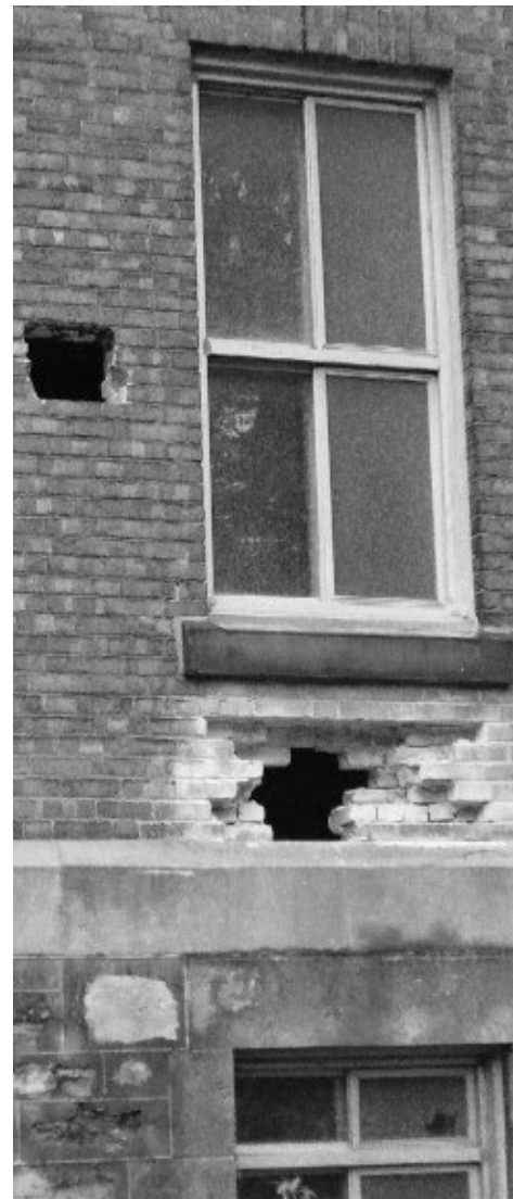
Two of the exploratory holes at 500 Claremont, as seen October 18, 2019.
