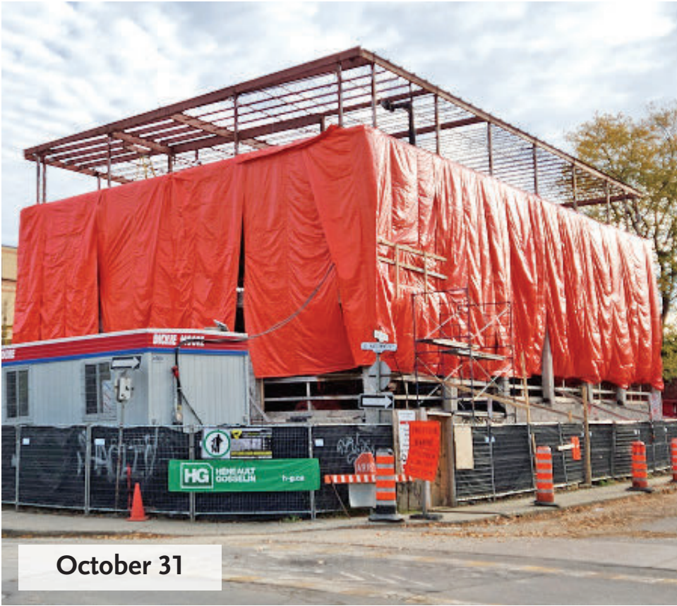
This existing building at St. Catherine and Prince Albert is being re-purposed into townhouses for the Albert Square project, as seen October 20, left, and October 31. It has been a skeleton for some time and the orange tarps were added between the time of these two photos, presumably to allow for winter work.
