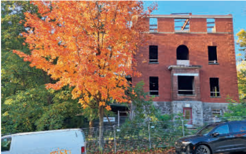
500 Claremont on October 21. The fifth floor, including its exterior brickwork (which was above the grey line), has been demolished and will be replaced (see January 18, p. 7). The building is to be rental apartments.
