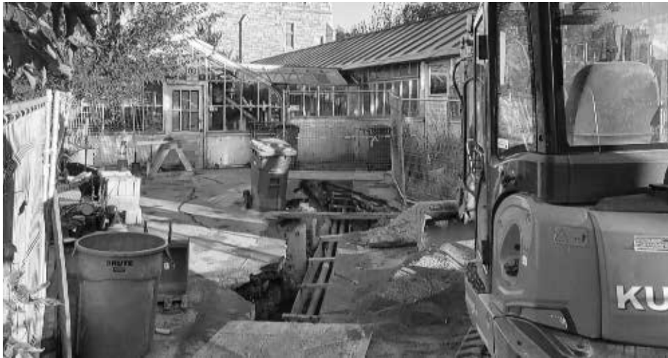
New underground electrical cables that will power the greenhouses, left, and dirt from digging work, as seen September 3 south of the work greenhouses.
