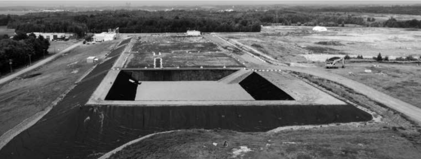
Sorted material is dumped into pits and then sealed with a membrane, as seen July 25.
