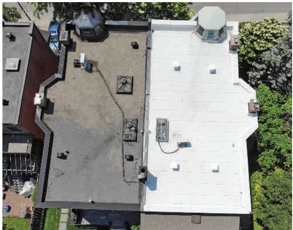
Two Arlington Ave. roofs were photographed June 7 using an infrared camera: one black measuring 57°C, left; one white measuring 46°C. The government of Canada's website puts the maximum temperature for Montreal that day at 32.3°C.
