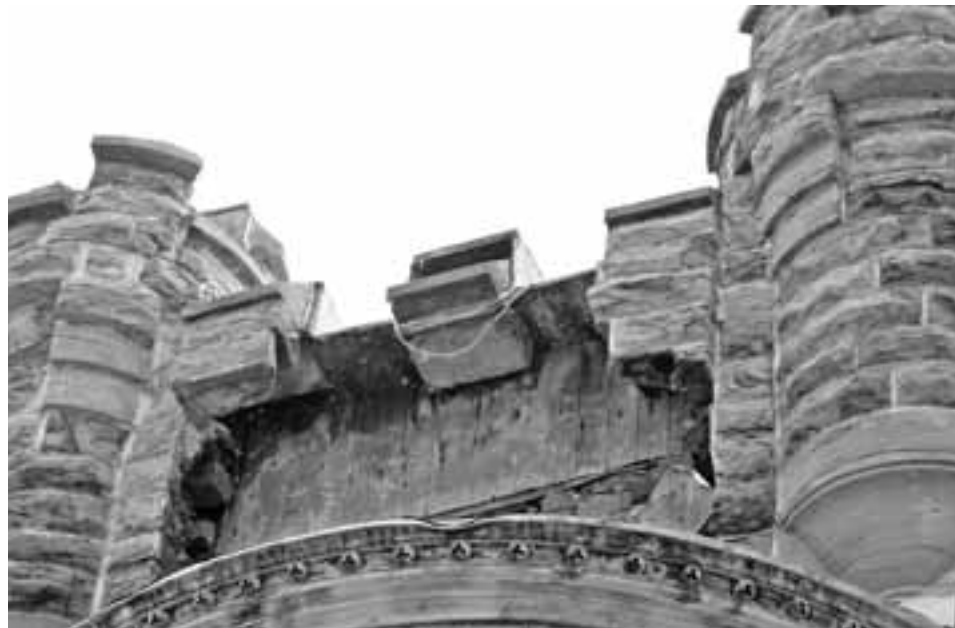
This deteriorating brickwork on the upper façade of 4030 Dorchester Blvd. on March 6.
