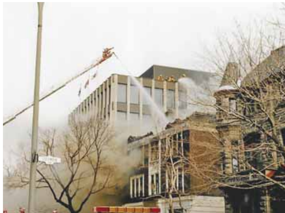
The original apartment building was destroyed by fire April 25, 1999.
