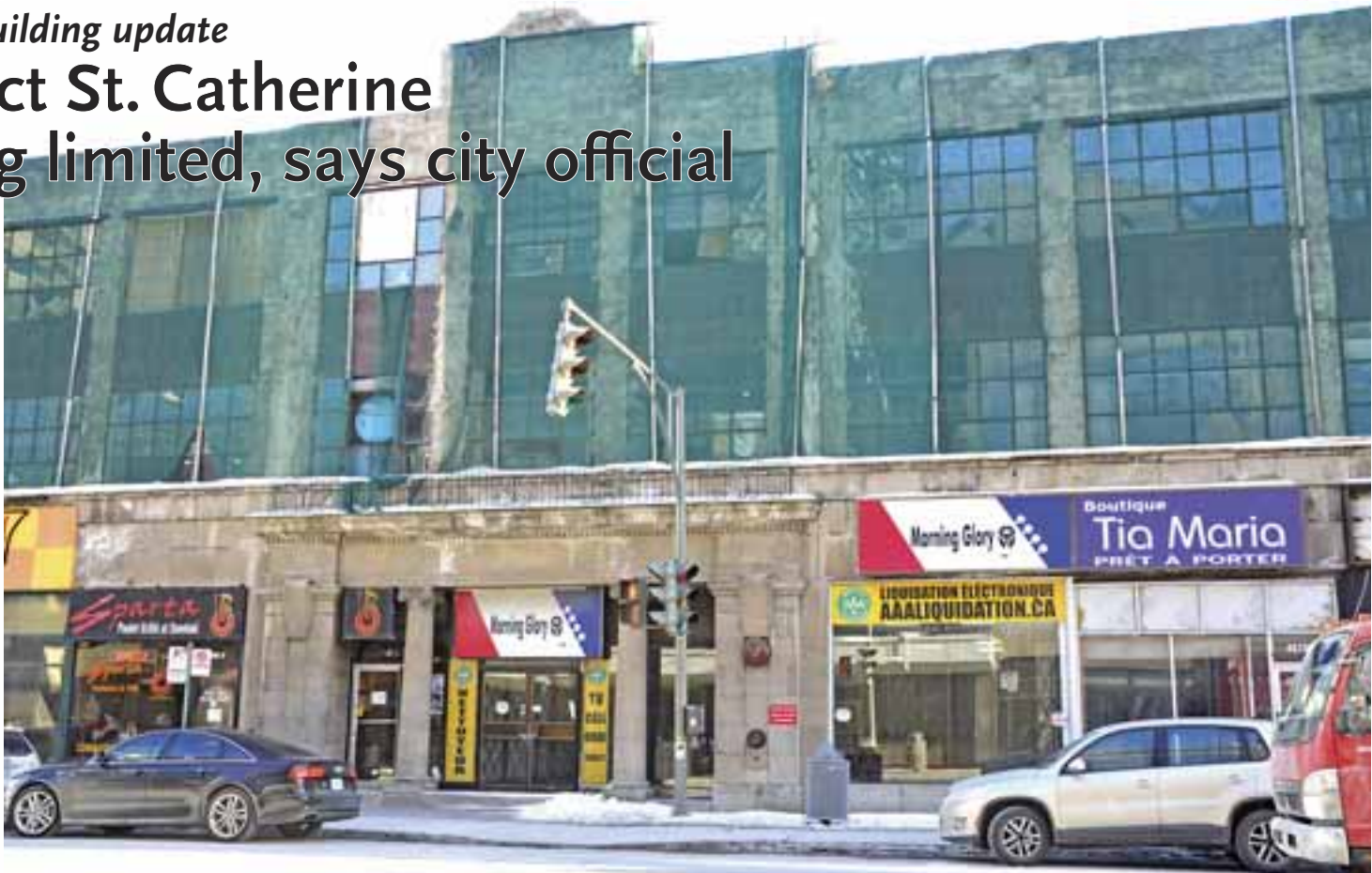
Most of the facade of 4026-32 St. Catherine has been removed and a protective screen has been placed over the building’s front to keep anything left from falling off.
