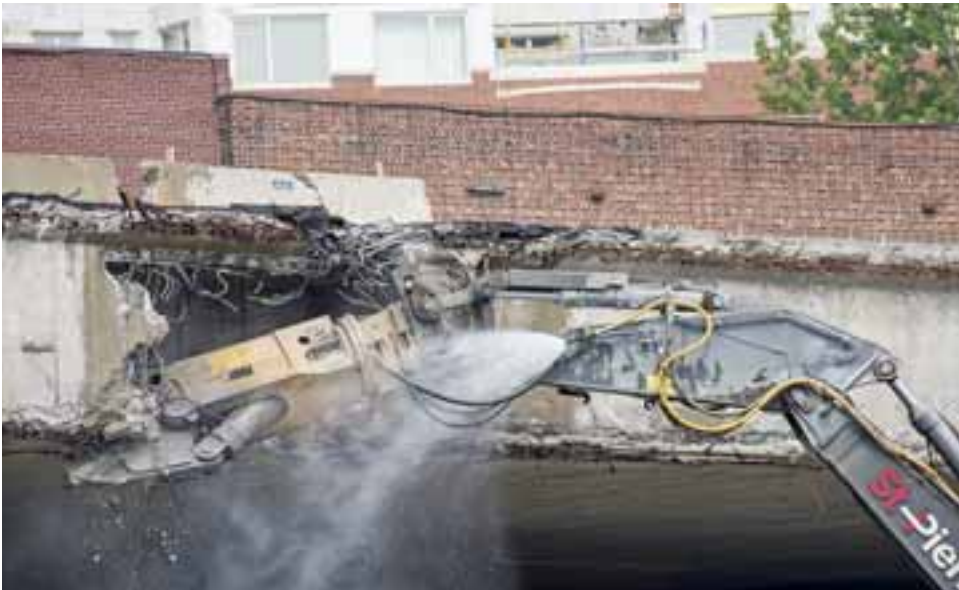
As mooted at the August 22 Bon Voisinage meeting, the KPH-Turcot construction consortium was using water cannon attached to these scissors on August 25.
