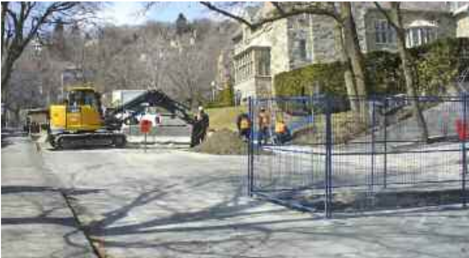
Workers continue installing public water service entries on the east side of Argyle south of Westmount Ave. April 9.
